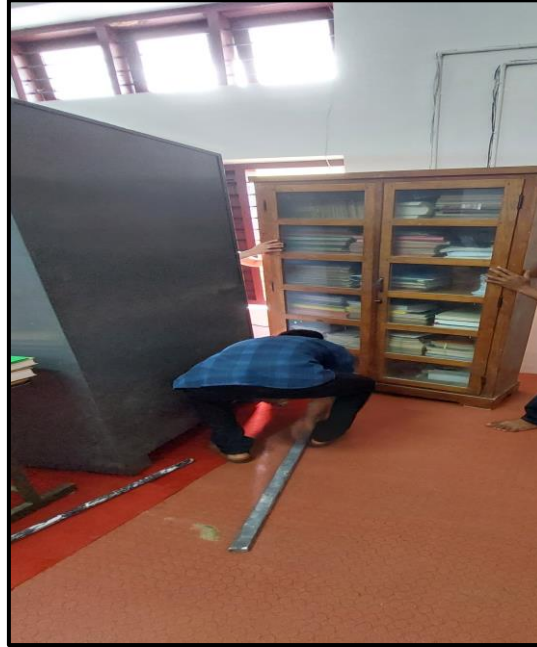
Renovation works done at the library
