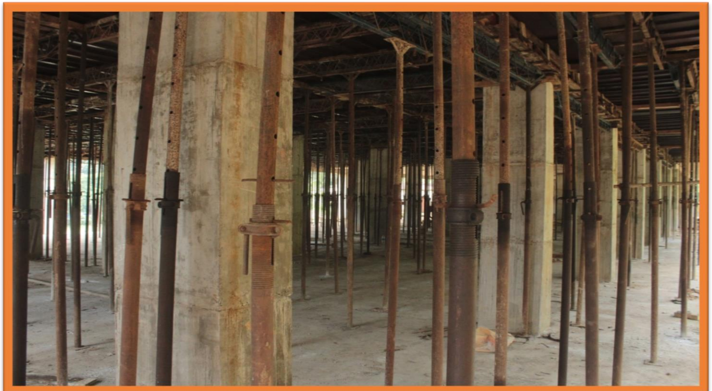
New Administrative Block under Construction
