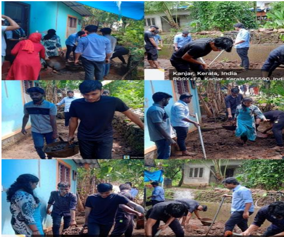
Cleaning Initiative at Kudayathoor: land-slide hit area community intervention
